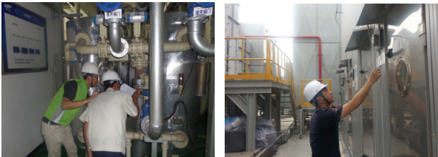
On-site inspection of utility facilities On-site inspection of environmental facilities
